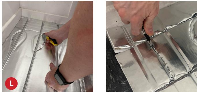
Start laying the pipes from the manifold, leaving enough slack for connection to the correct port. It is recommended to use a pipe decoiler when laying especially when one individual is available. The decoiler keeps the piping system organised and prevents tangling or kinking during the installation process.
