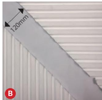
Where there is a corner with high pipe density it can be formed from a transitional board. Cutting two opposite 45° sections will provide a 90° turn **B**. A gap of 120mm wide should be left to allow the pipe to curve smoothly. Fill this area using a self leveling mix apply to the level of the overfloor boards.
