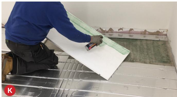
The 500ml spray can be set to three positions - LOW, MEDIUM & HIGH, indicated L, M, H. We recommend setting the spray between M & H.
