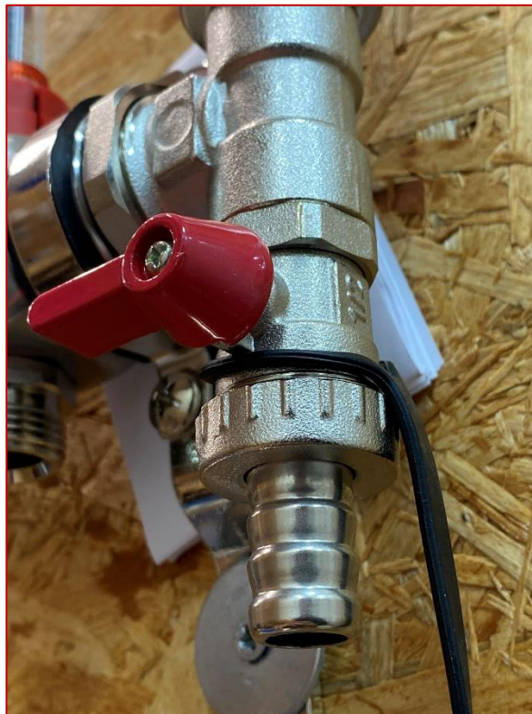
Fig. 12.3 (above) - Hose union fitted in place of end caps.
