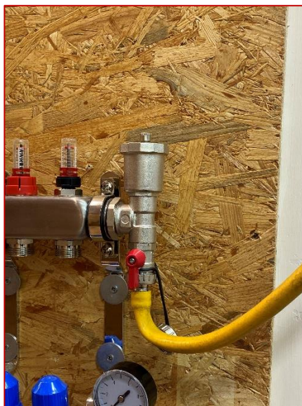
Fig. 14- Hoses connected to the flow (left) and return (right).
