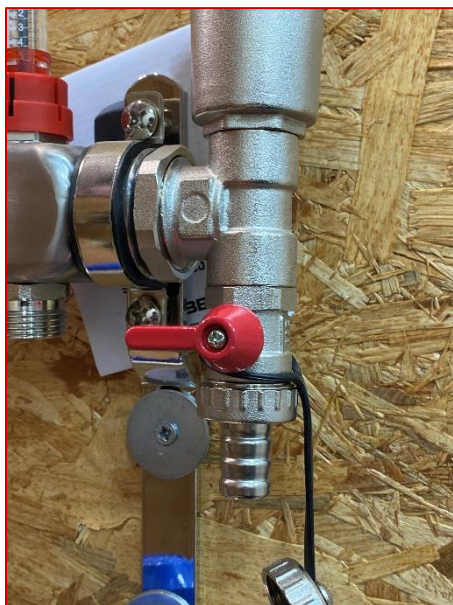
Fig. 13.1 – Valve on air vent assembly in the closed position.
