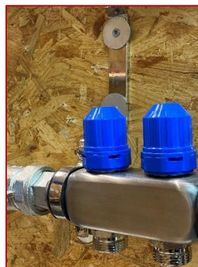
Fig. 15.1 – Flow valve (left), shown with the locking cap attached and removed. Once removed, the black part can be twisted.
