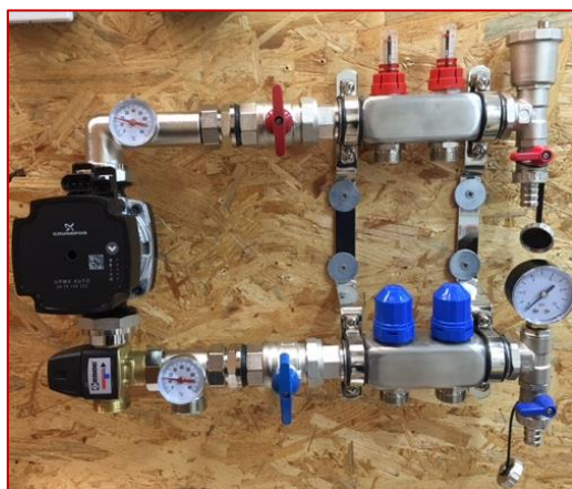
Fig. 4 – Manifold with control pack fitted (left; black units with temperature gauges).
